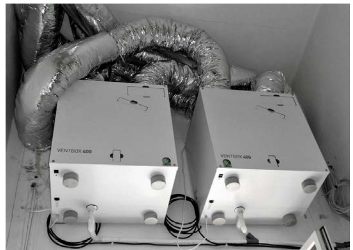
Two ventilation units with heat recovery (VENTBOX 400)
