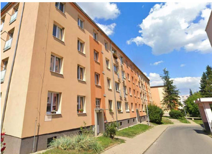
One of the affected residential buildings
