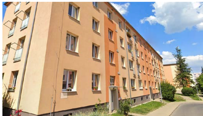
One of the affected residential buildings
