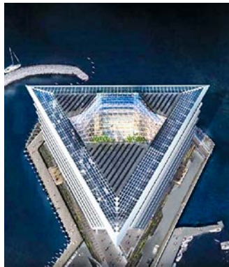
Ferring, Copenhagen, Denmark
