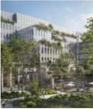
UBS Pleyad Business Centre Saint-Denis, France
