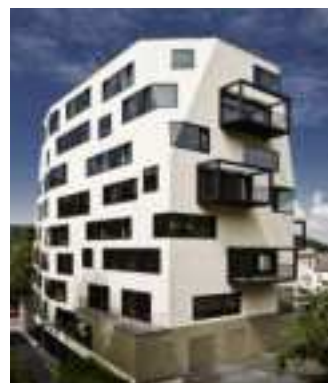
Triplex – Apartment block, Karlovy Vary, Czech Republic
