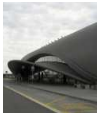
Airport, Brno, Czech Republic
